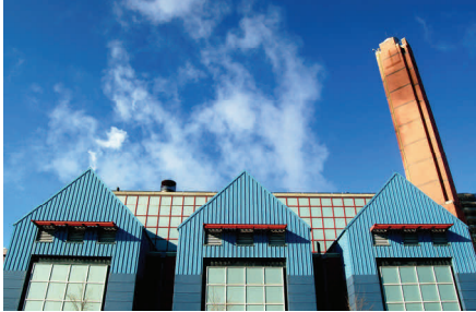
Abstract photograph of the Central Utility Plant, 2009
