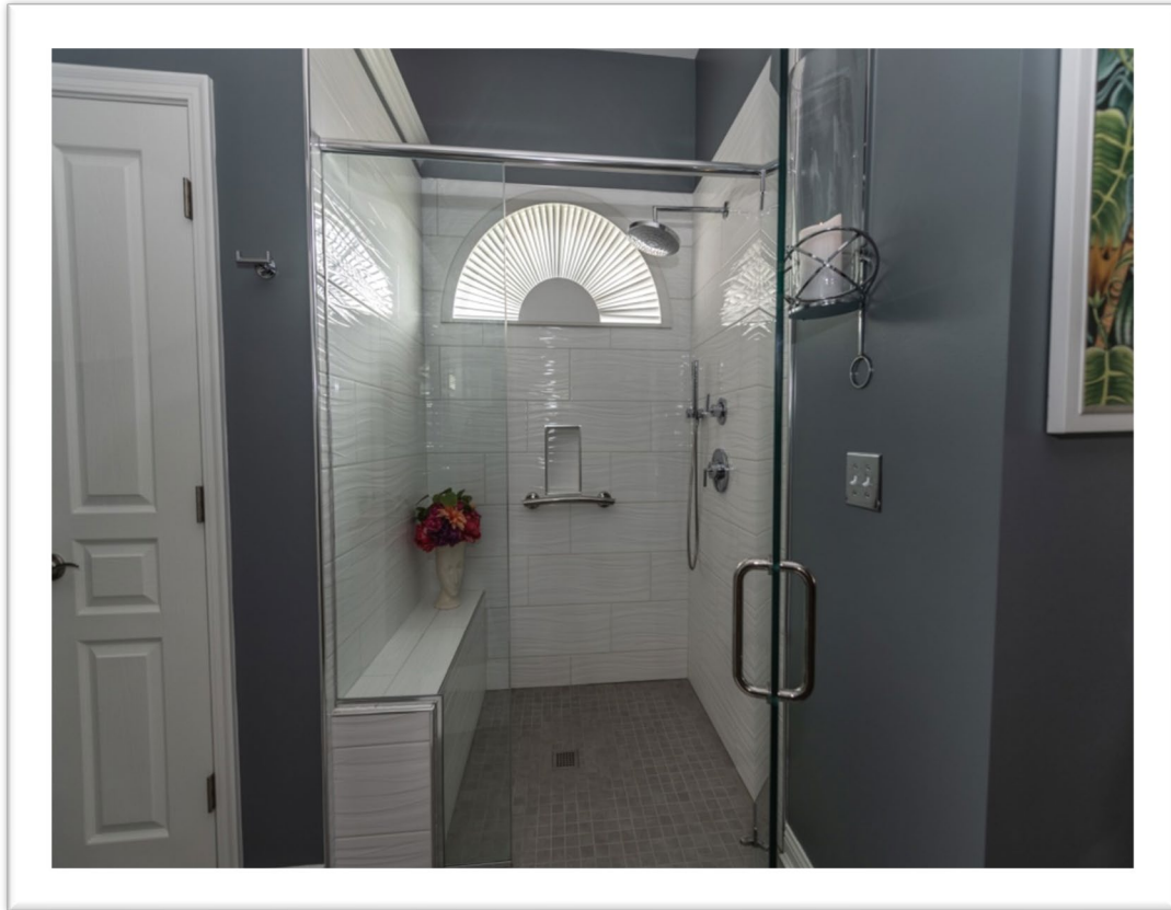
Full room remodel with barrier-free shower
